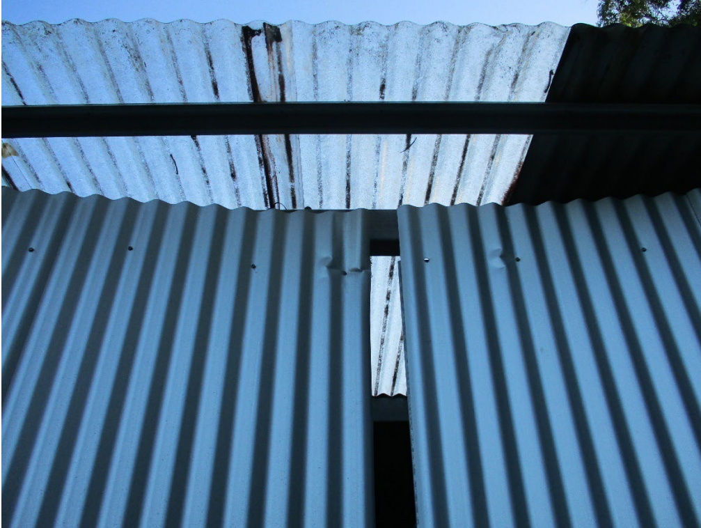
Photograph 8 Wall and roof of a corrugated iron shed with noticeable gaps
